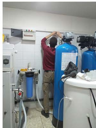
INSTALLATION OF A NEW WATER TREATMENT SYSTEM AT HAMSHARI HOSPITAL HEMODIALYSIS CENTER
